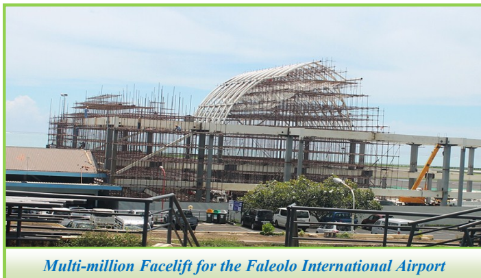
Figure 1: Faleolo International Airport work in progress
